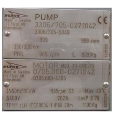
Serial number 3306/705-0271042 3306/705-5049 Product number **Approvals** CF Curve number 53-610 Voltage 400 V Current 202 A **Delivery connection** Rated power, shaft 100 kW Input power 109 kW Cos phi 0,78 Weight 1520 kg
